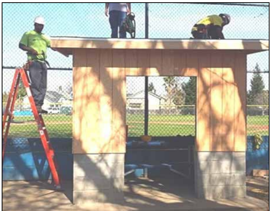
NCCT works on the construction of a CGLL score booth
