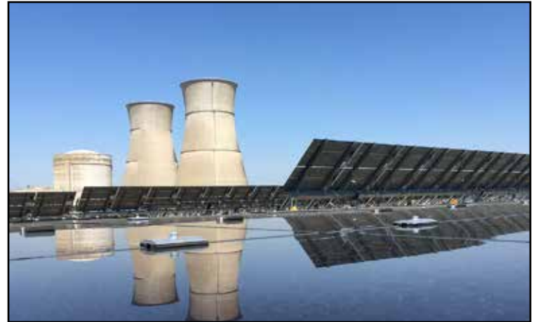
Solar panels at Rancho Seco.
